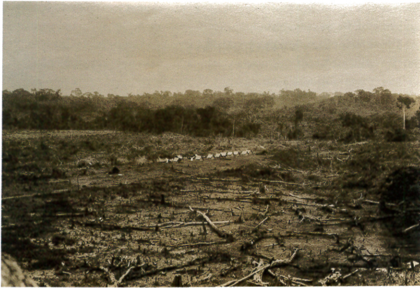
FIGURE 6.1. Large-scale clearing for the Firestone plantations, capturing a “birds-eye view” of a landscape in transition. Loring Whitman. 6 August 1926. Courtesy of Indiana University Liberian Collections.
